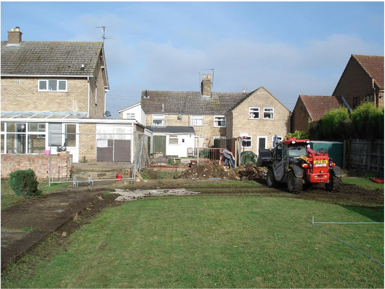
General view from dormer window position towards Mill Road.
